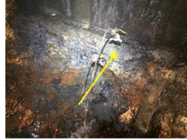
Drilled Hole with Packer
