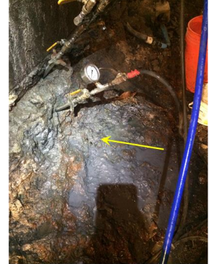
NOH2O Sealing the Leak
